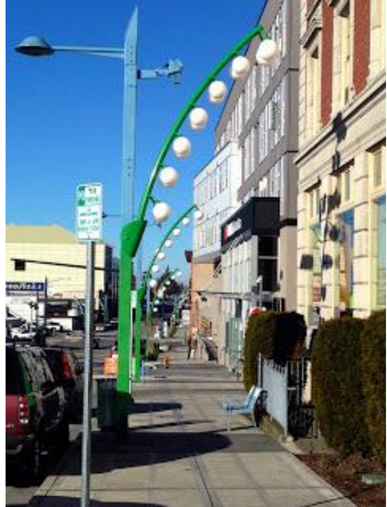
Artspace Everett Lofts, Everett, WA
