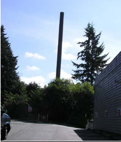
Acceptable Monopole WCF
