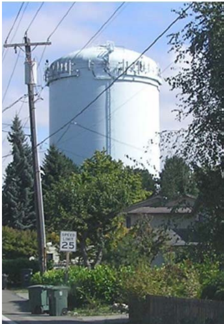
Acceptable Structure-Mounted WCF
